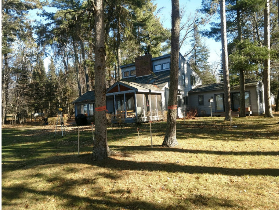
Staked 10' x 25' rockbed facing East. Marked trees to be cut at grade with stumps in place by homeowner prior to installation
