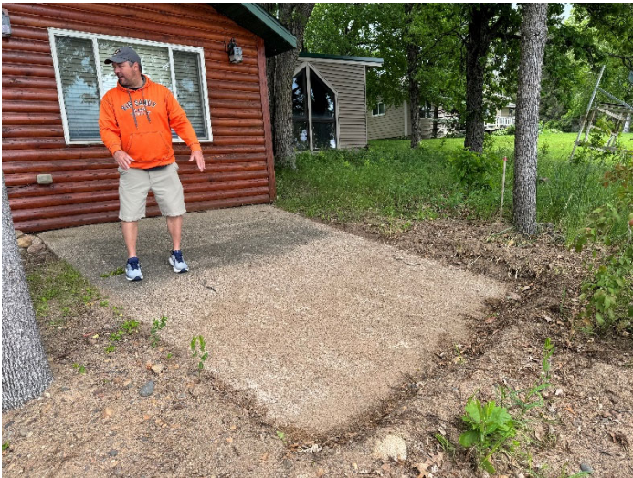
Installer to crush and remove concrete pad
