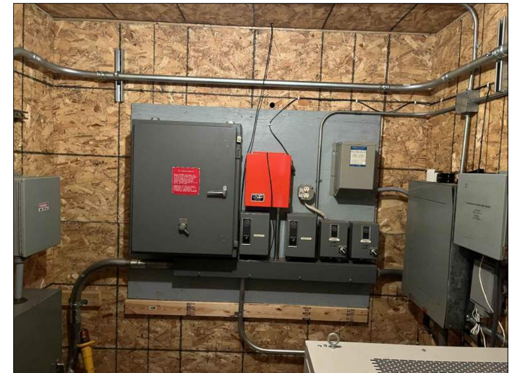
EXISTING VAULT INTERIOR
