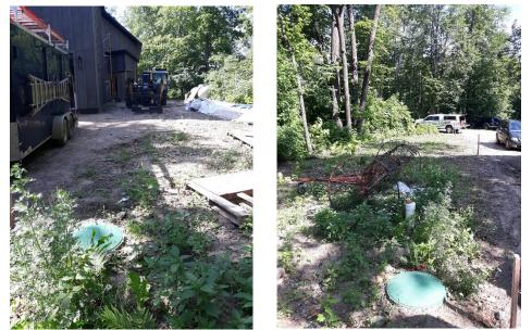
Existing tank looking towards the cabin and from the cabin down driveway. This tank will be pumped, crushed, and removed. The new tank will be set in its place
