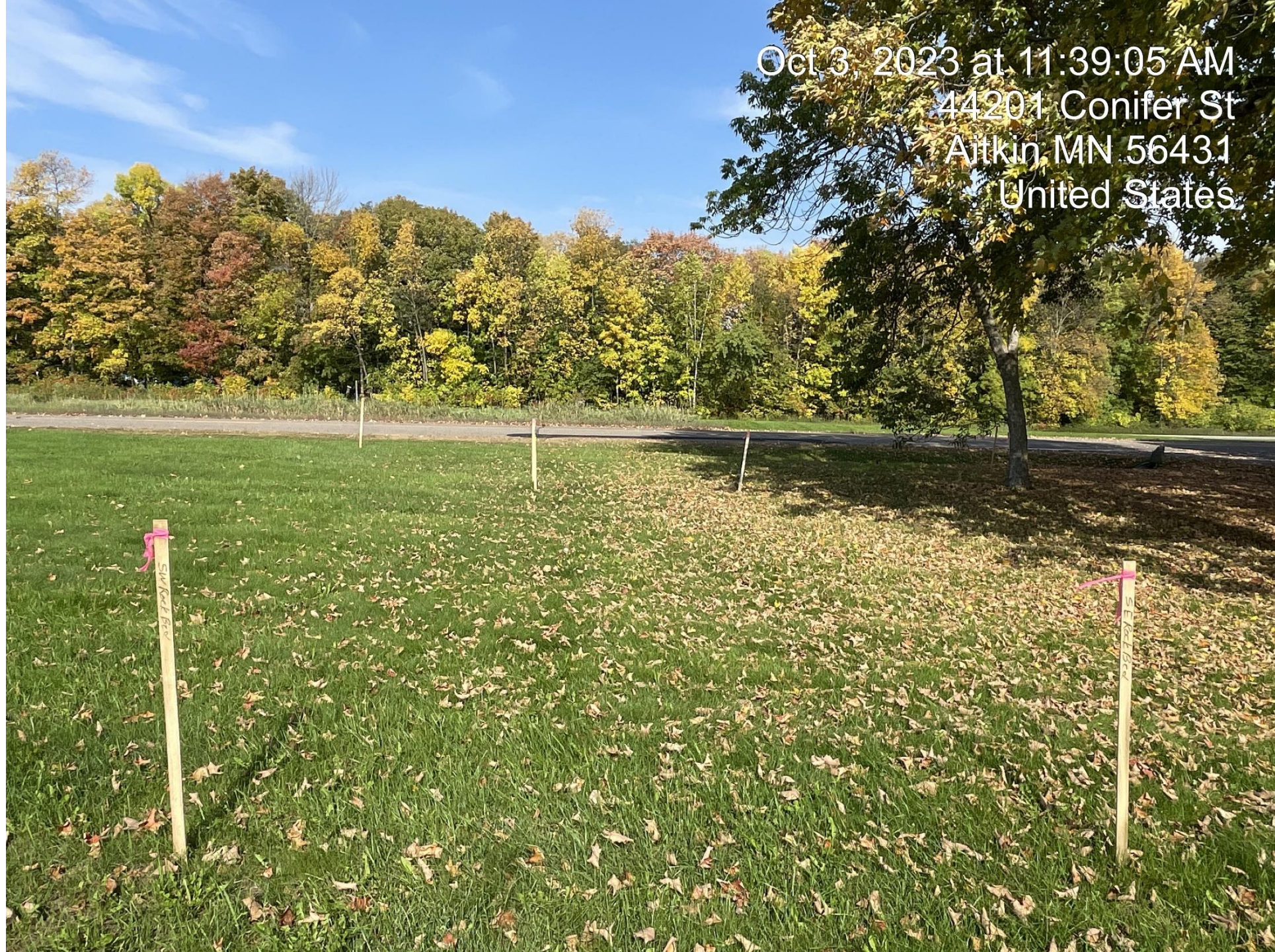
Type 1 Mound Septic Rockbed
