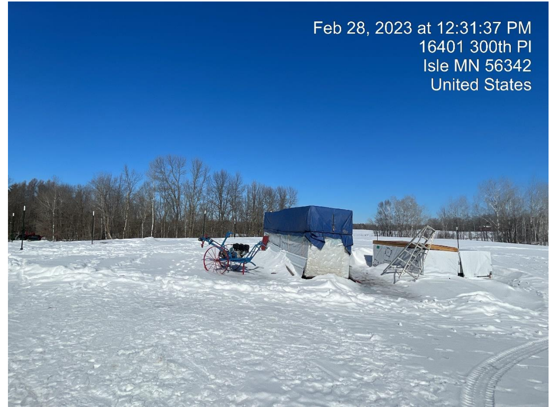
House staked out
