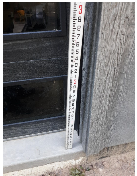
Benchmark on Concrete at garage door.
