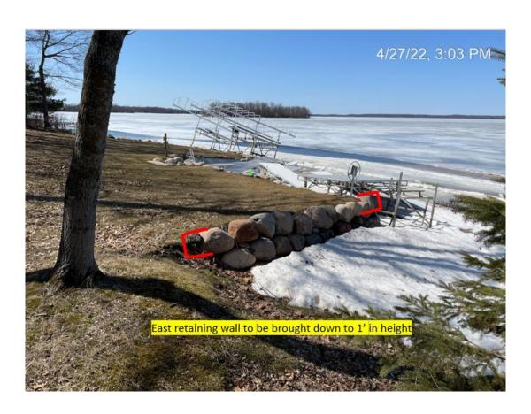
Retaining walls to be placed in pre-existing location with measurements as indicated on image below.
