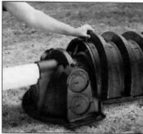
2. Place first chamber onto endcap.
