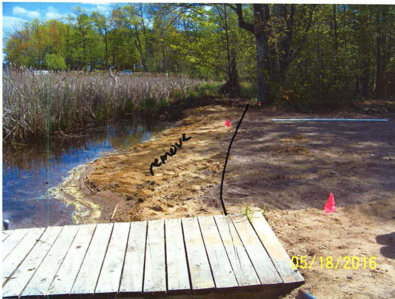
Another view of the fill removal area.
